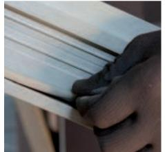
leaf opening direction. Verify that the sealing strips are inserted in the suitable seats present in the aluminum facings (1 horizontal + 2 vertical).
