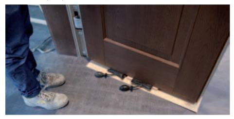
Close the door and verify that the leaf is centered with reference to the frame opening. Correct any differences by acting on the adjustment points.
